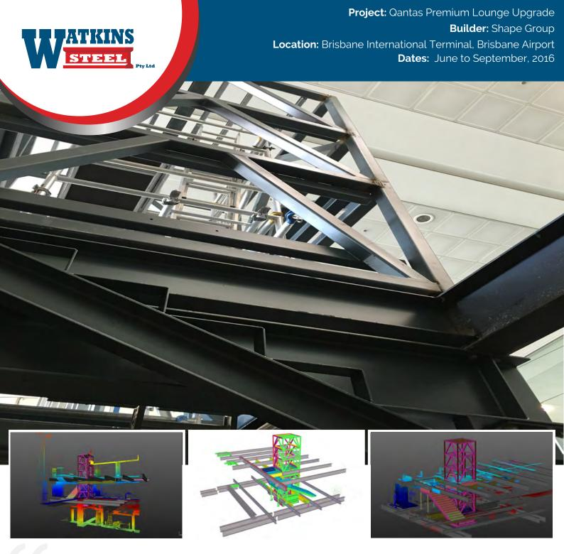
The biggest challenge for this project were the complex geometric dimensions through three different levels. Using the 3D laser scanner with the RTS total station we were able to produce an accurate existing model to overcome this challenge. The result being that the project was delivered a week ahead the construction schedule with zero rectification works.
