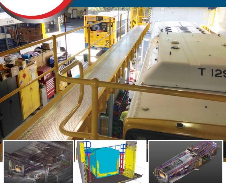
Combining the use of the laser scanner and total station with Tekla modelling gave us peace of mind that the steelwork would be spot-on. Designing and installing a tight-fitting maintenance platform meant there was no margin for error. It was great seeing the first bus roll into the bay—it fit perfectly.
